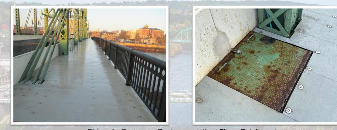
Sidewalk System: Replace existing Fiber Reinforced Polymer (FRP) sidewalk decking with new closed-cell FRP panels spanning from panel point to panel point, including new access hatches with tie-off provisions, and cutouts in panels at truss components and railing posts.
