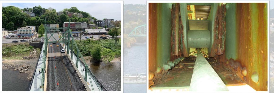
Painting of superstructure: Replace paint system by installation of working platforms and necessary containment, removal of existing paint system through blasting with additional attention at panel points, and re-painting with 3-coat organic zinc paint system. Includes detailed light color painting within verticals, finials, and cross struts at piers. Also includes waste disposal, worker health and safety, and environmental protection measures.
