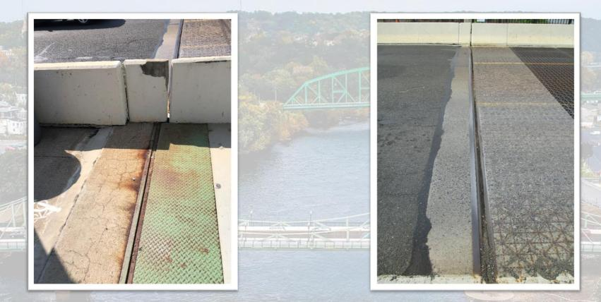
Joint Replacement: Reconstruct the joints at abutments by demolition and replacement of the sidewalk headblock, partial removal of roadway barrier for connection of the upturn to the existing roadway joint extrusion, installing of a continuous neoprene seal across the width of the bridge, rebuilding of the roadway barrier, and replacement of the sidewalk plates.
