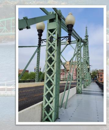
Ornamental Highway/Sidewalk Lighting: Replace existing lighting fixtures with LED fixtures, supports, conduit and wiring.
