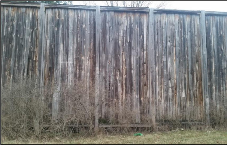
Existing Noise Walls on I-95 Southbound (To Remain)
