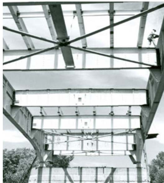
▲ The Scudder Falls Bridge under construction in 1959; its non-redundant design was similar to the Mianus River Bridge that collapsed in Connecticut in 1983.
