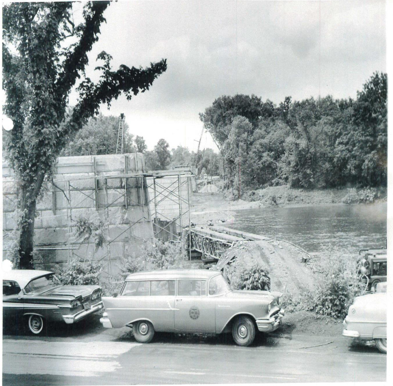
Figure 4. Construction of SFB in 1959; view from New Jersey toward Park Island.
