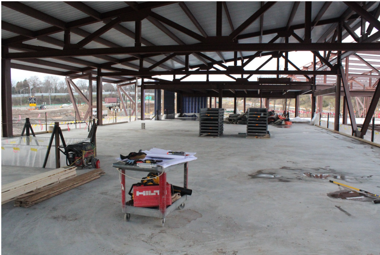
Steel Erection and Slab on Deck
