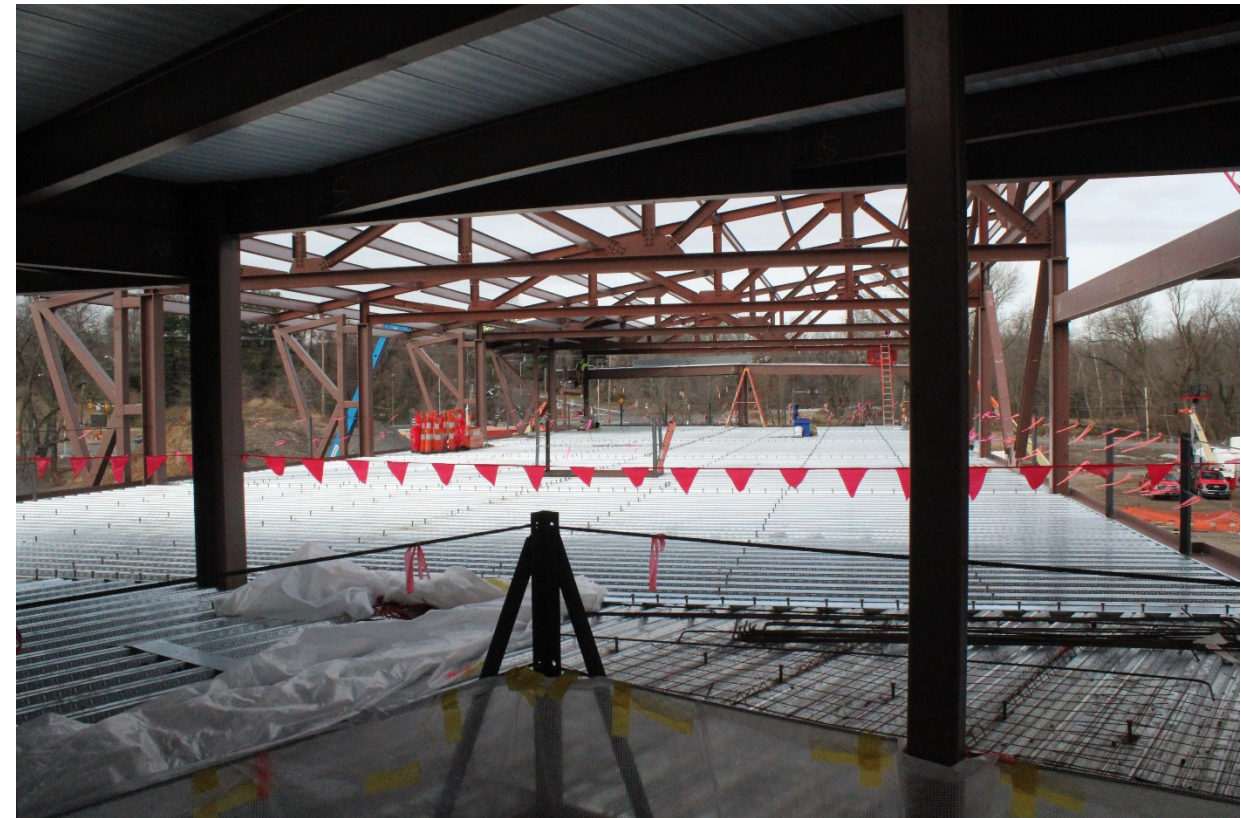
Steel Erection and Slab on Deck
