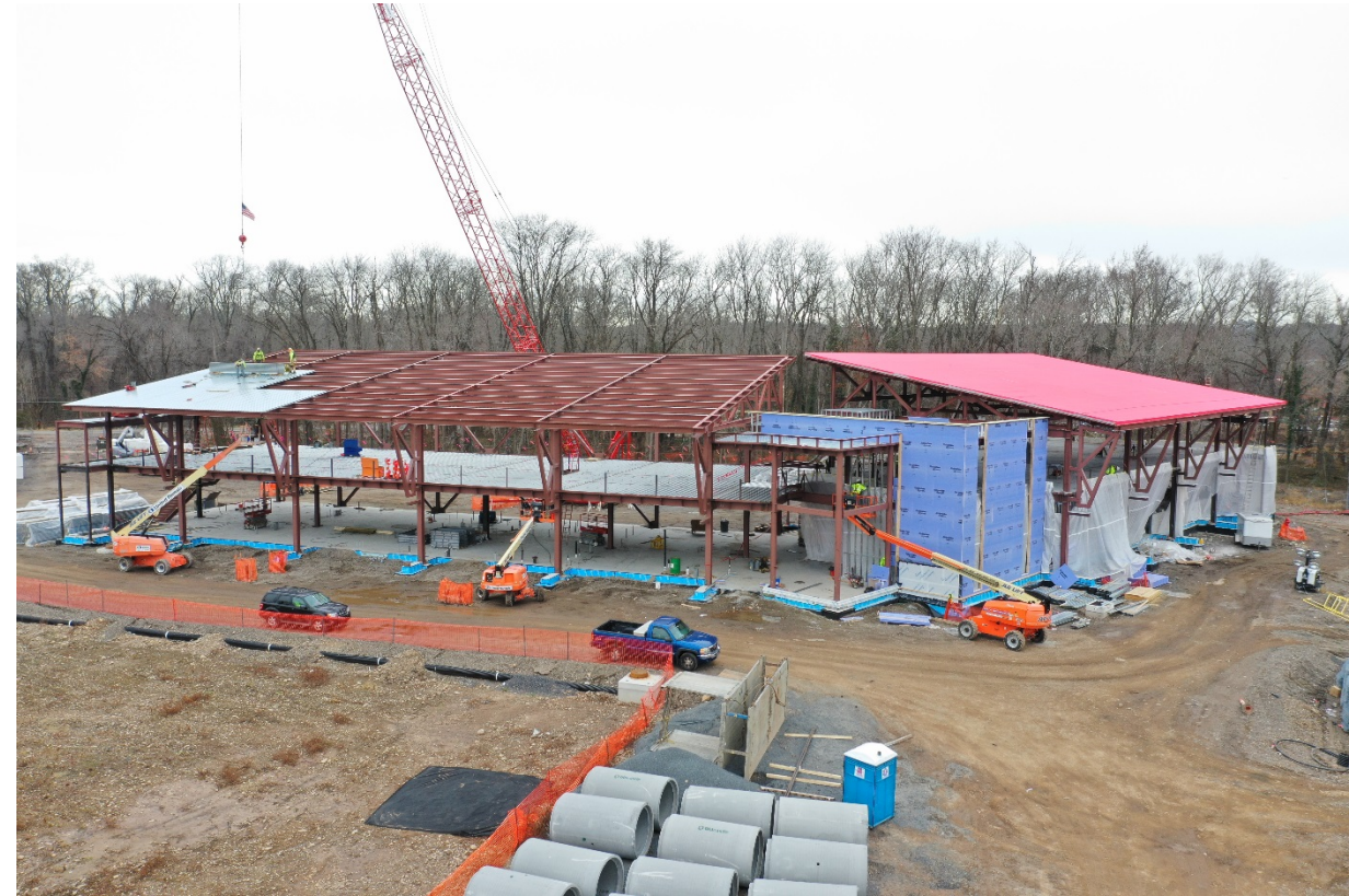
Steel Erection and Curtain Wall
