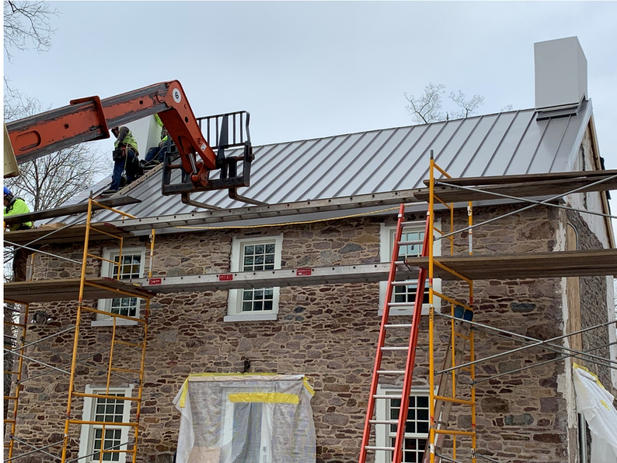
Roof Installation
