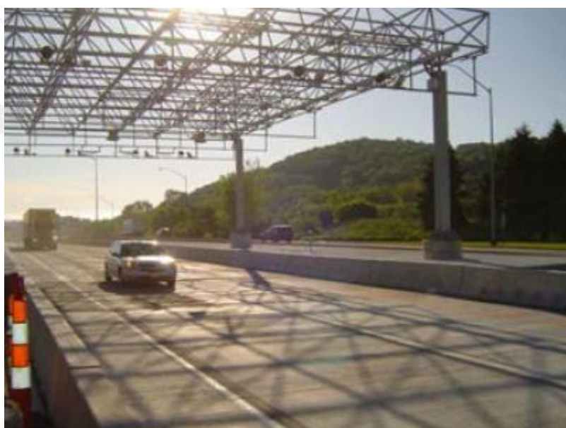
Figure 3—Example Overhead Toll Gantry (Space Frame) on I-78 in PA
