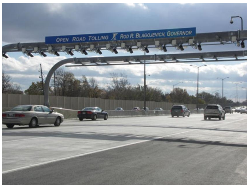
Figure 2—Example Overhead Toll Gantry, Monotube Design, Illinois Tollway
