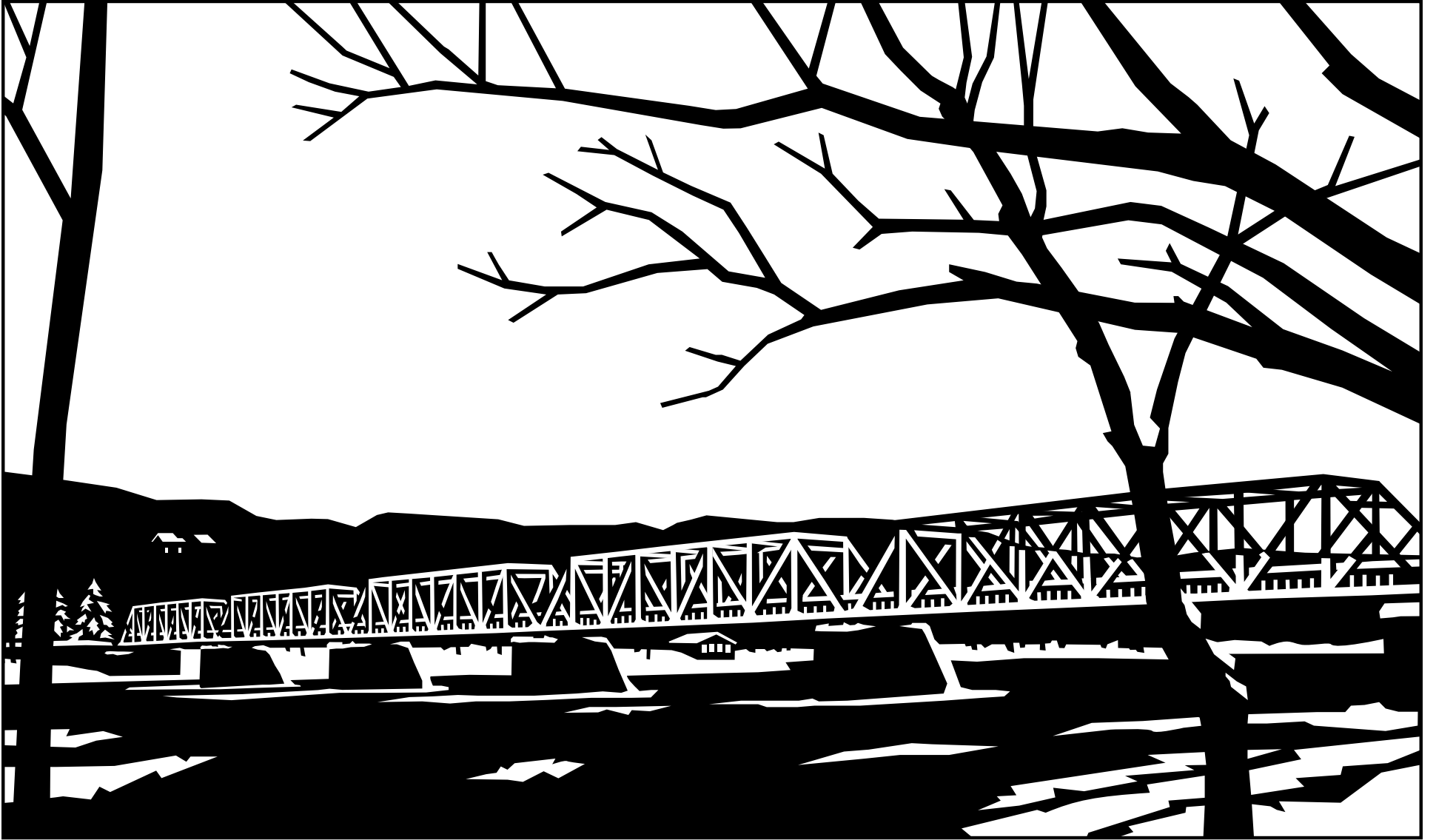
▲ Uhlerstown-Frenchtown Toll-Supported Bridge
