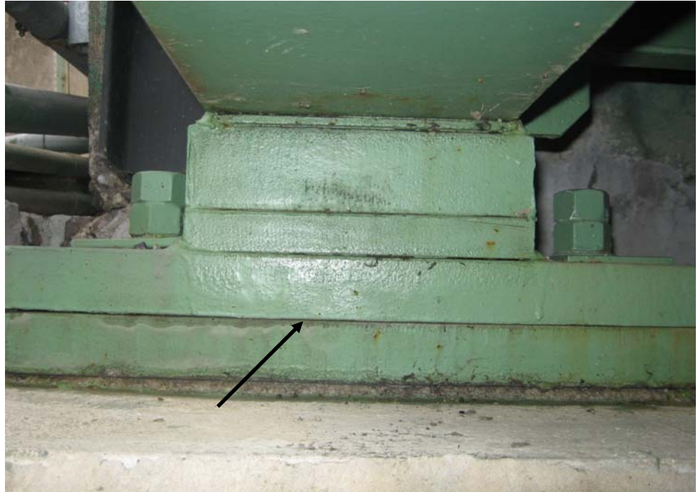
PHOTO 1 General view of the south fascia sidewalk stringer bearing, looking west. Note there is no sliding plate or gap between the masonry plate and sole plate.
