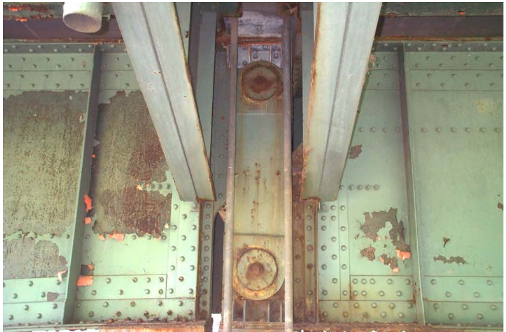
PHOTO 6 General view of the pin and hanger assembly (North girder at Span 1 shown), looking south. Note the light to moderate rust throughout assembly and seismic retrofit.
