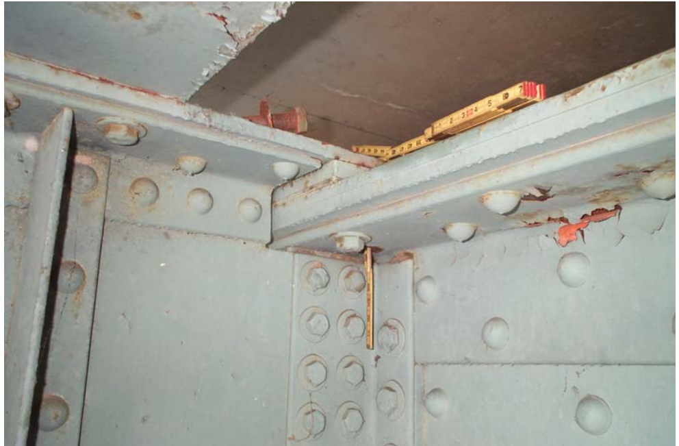
PHOTO 5 1 of 8 connection bolts is sheared at the tie plate connection over the north girder at the first floorbeam to the east of Pier 8, looking east.
