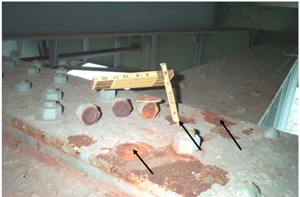
PHOTO 4 3 of 8 connection bolts are sheared at the tie plate connection over the north girder at the floorbeam at Pier 8, looking west.
