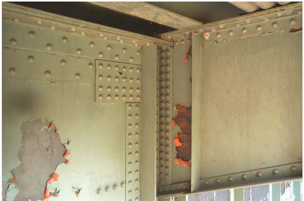
PHOTO 2 Typical Cantilever bracket (Floorbeam 3 at Span 1 shown), looking northeast.
