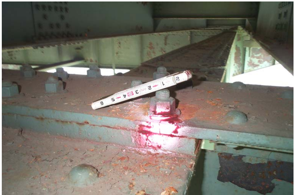
PHOTO 3 Crack in the tie plate over the south girder at the first floorbeam east of Pier 5, looking east. The crack is arrested by a tie plate connection bolt hole and there are no signs of crack propagation.
