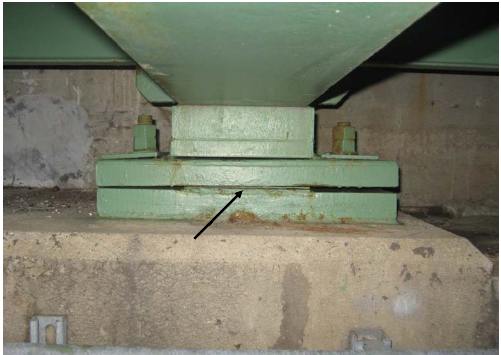
PHOTO 2 General view of the Sidewalk Stringer 2 (from south) bearing, looking west. Note the sliding plate between the masonry plate and sole plate.
