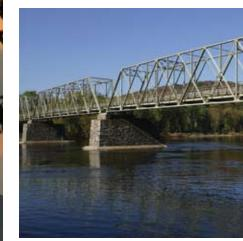
The existing bridge, constructed in 1904, is a four-span, riveted steel, double Warren truss structure, with a total length of 653 feet. The steel open-grate deck provides a clear roadway width of 16 feet between tri-beam railings. In addition, a concrete-filled grating sidewalk is supported on the upriver truss with steel cantilever brackets.
